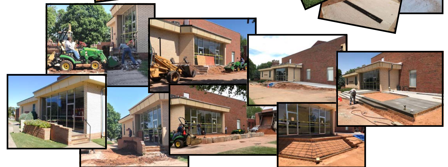
Renovation of the west side of the Student Center had been planned for last summer, but did not happen. Plans are to replace the broken concrete that runs from the west side of the building to the north side of the science building. So much student/guest/employee traffic happens in this area, the work was needed to improve the area's
