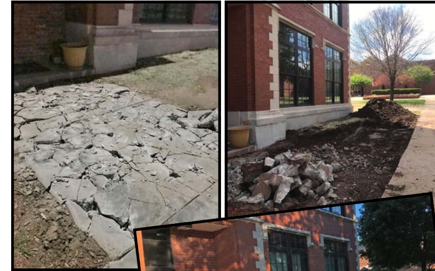
This past spring some work was done on the west side of Ryerson Hall, adding a much needed parking pad for the Student Services golf cart. The next sidewalk project will be replacing sections of the sidewalk around the building.
