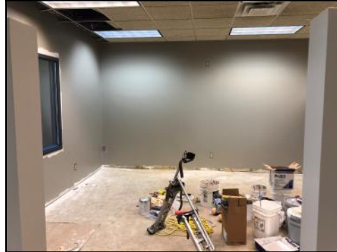
Construction is underway at the new VR lab. Projected completion date is August, 2019.
